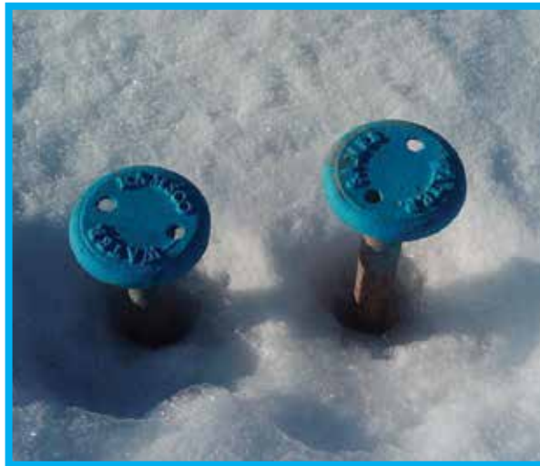
Above: A curb box or curb stop can be marked with blue paint
