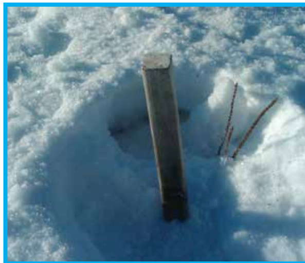
Below: If a curb stop is in the ground, a wooden stake is a good marker
